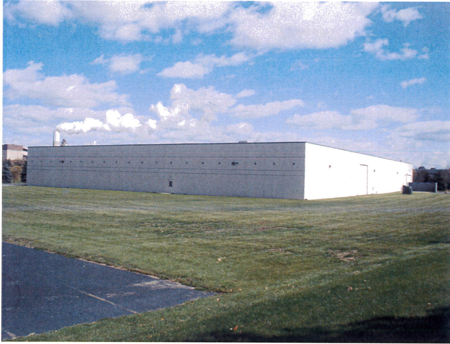
Southwest corner of building; camera looking northeast (View from Fair Oaks Farms)
