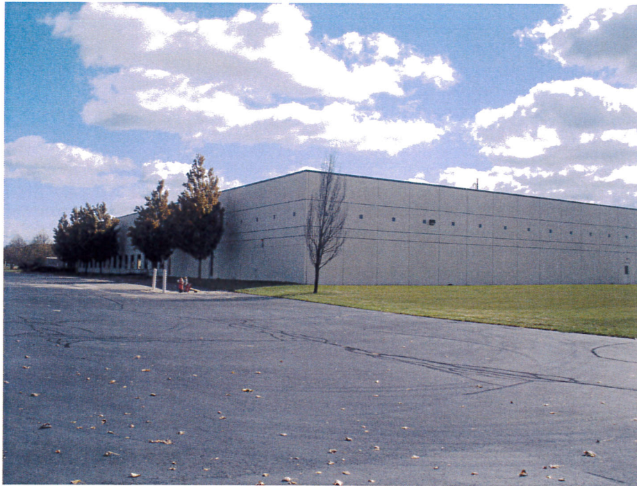
Northwest corner of building; camera looking southeast
