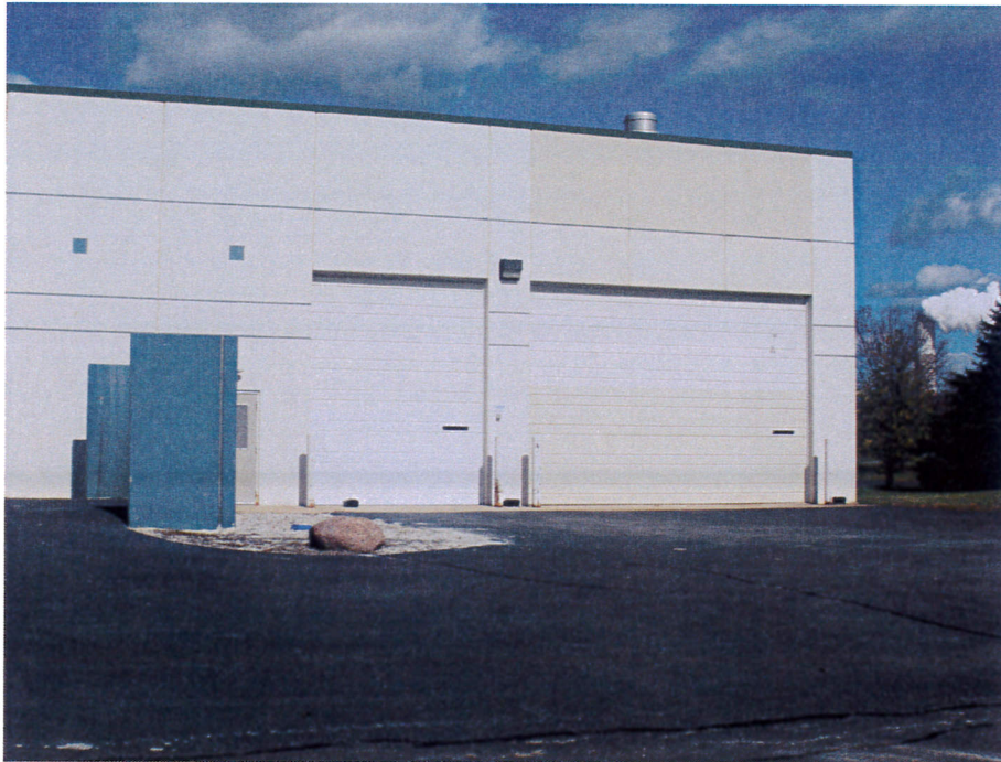
Eastern face of South Elevation; camera looking North (Loading dock area and dumpster screen)
