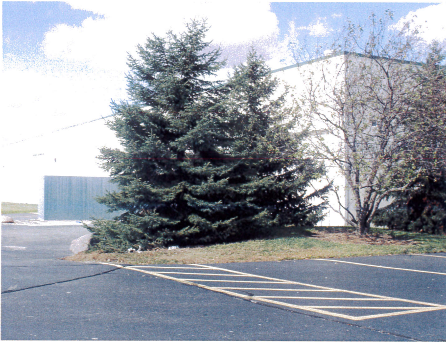
Southeast corner of building; camera looking northwest (Loading dock area and dumpster screen)
